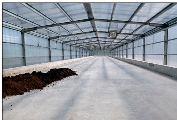
**Figure 1.** Solar drying greenhouse of the Areias de Vilar WTP.
