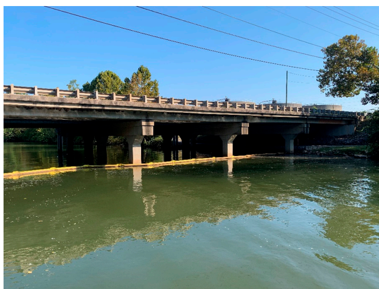
Figure A1. Deployment of the spill containment boom (yellow) across the confluence point of Third Creek and the Tennessee River.
