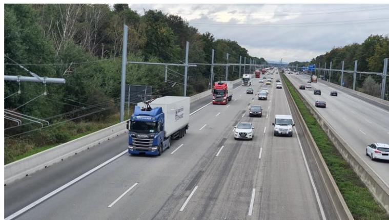
**Figure 1.** eHighway system in Germany (IVV, 2021).
