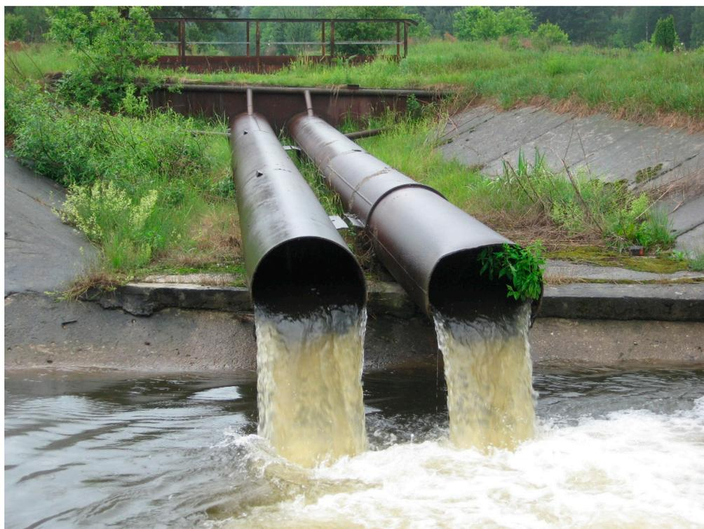
**Figure 2.** Discharge of brown coal mine waters treated in settling ponds.
