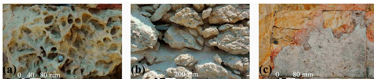
**Figure 1.** Degradation forms of the Calcari di Cagliari limestones: (a) alveolization of the Pietra Cantone; (b) loss of material and pulverization in a wall built with Tramezzario ashlar; (c) detachment and oxidation in a Pietra Forte ashlar.
