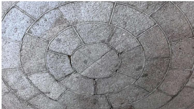
**Figure 12.** Detail of vault centre, with keystone formed by two symmetrical voussoirs (photograph by author).
