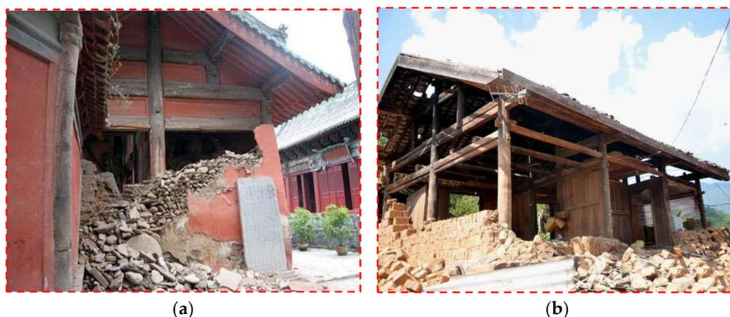
**Figure 1.** Common seismic damages to the walls in traditional timber residences. (a) Local collapse of the wall; (b) overall collapse of the wall.
