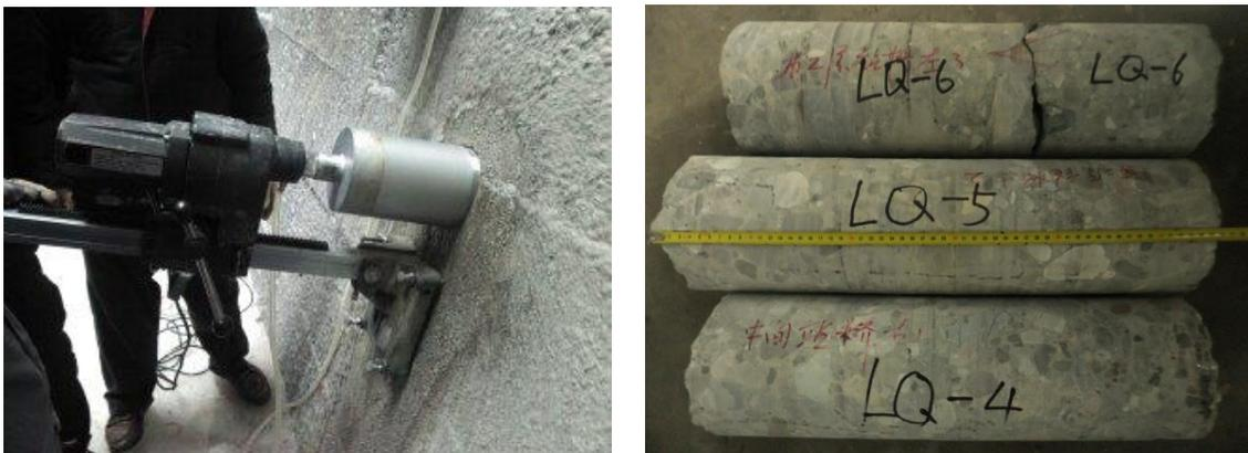
**Figure 3.** Illustration of on-site core sampling.
