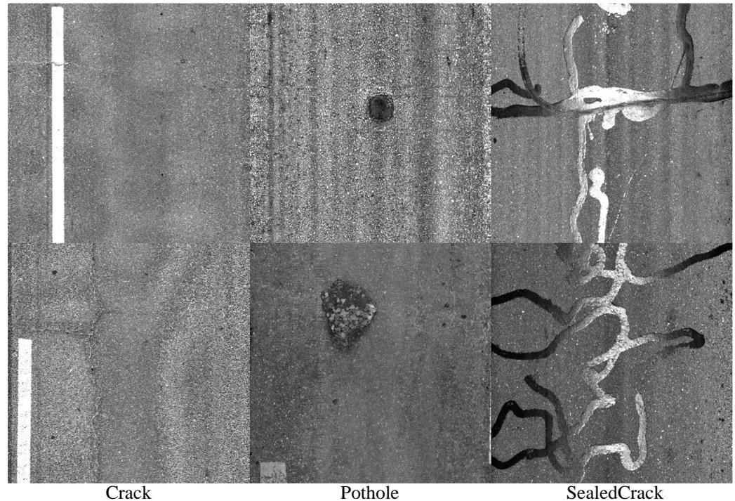
**Figure 5.** A sample of pavement distress types.
