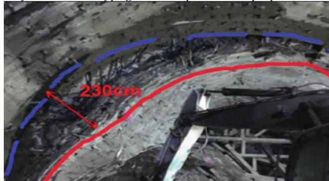
(b) Large deformation of the local vault in Muzhailing Tunnel.
