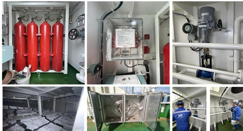
**Figure 13.** Prototype test (above) and target ship installation (below). Third-party verification certificate (below right) of the BSS.
