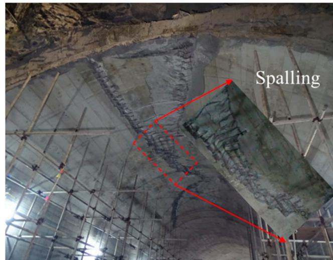
**Figure 10.** Blasting-induced spalling failure of rock mass in the access tunnel.
