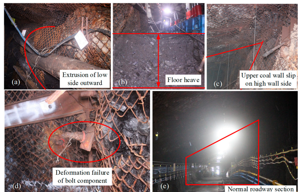
Figure 11. Deformation and failure characteristics of surrounding rock of right-angle trapezoidal roadway on site.
