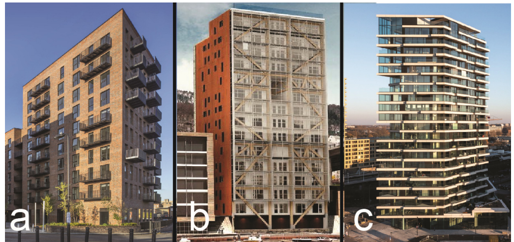
Figure 3. High-rise wooden residential buildings: (a) “Dalston Lane” building in London: height 33.8 m; CLT construction; (b) “The Tree” building in Bergen: height 49.0 m; CLT construction, Glulam; (c) “Haut” building in Amsterdam: height 73.0 m; timber–concrete hybrid construction (source: Internet, accessed 10 September 2023).
