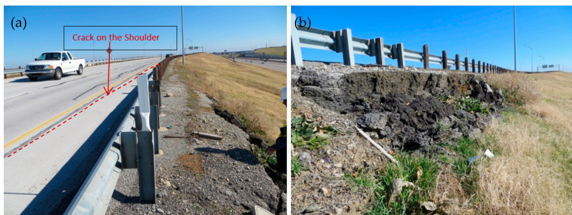
Figure 12. (a) Cracks on the shoulder; (b) failure at the crest of the slope.
